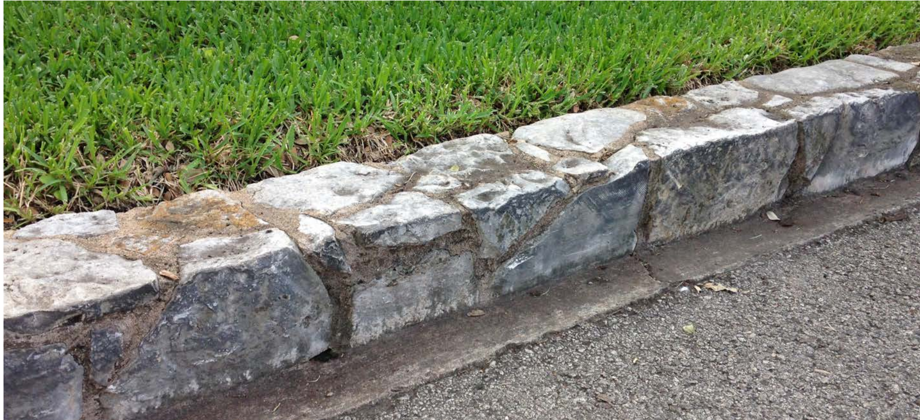
STONE CURB WITH GUTTER
