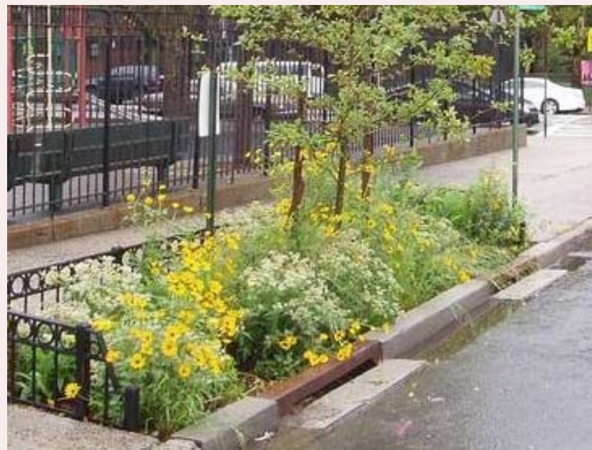
ARMORED CURB INLET
