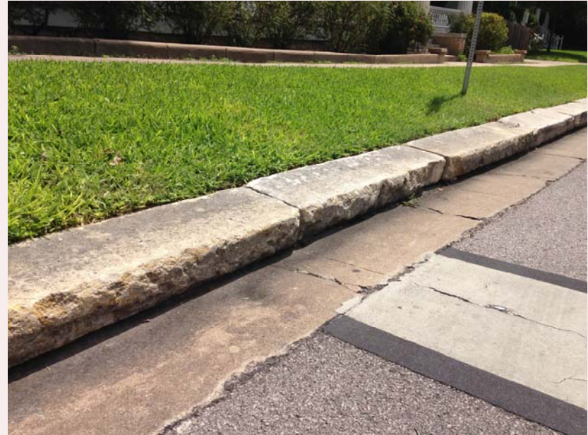
STONE CURB WITH GUTTER
