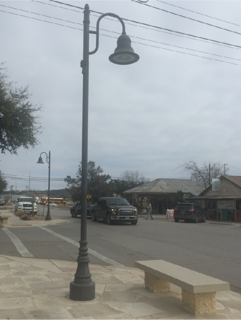
MERCER STREET LIGHTING
