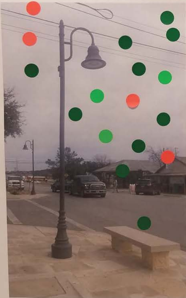
MERCER STREET LIGHTING
