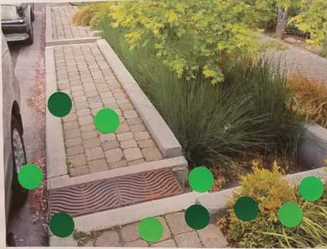
STRUCTURED RAIN GARDEN
