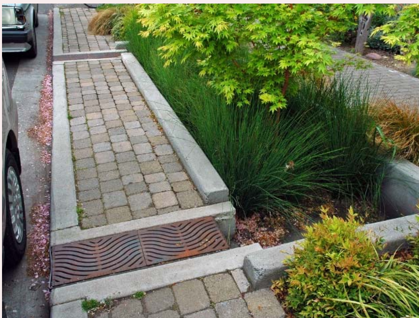
STRUCTURED RAIN GARDEN
