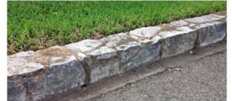
STONE CURB WITH GUTTER
