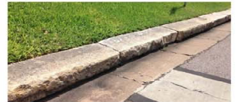
STONE CURB WITH GUTTER
